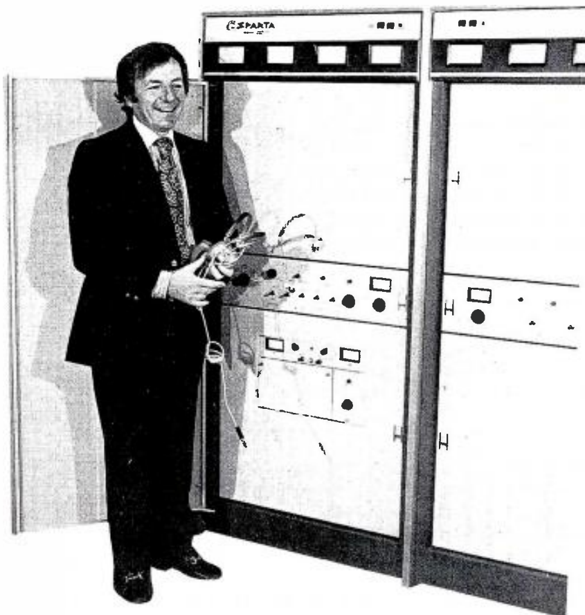
Mr. Ralph Guild, President of ASI Communications, Inc., shows his pleasure while inspecting the Sparta Model 620 FM Transmitter as installed at KFAC, Los Angeles. Other ASI stations include WERE, Cleveland; WRYT, Boston; KROY, Sacramento, KJTV, Bakersfield.
